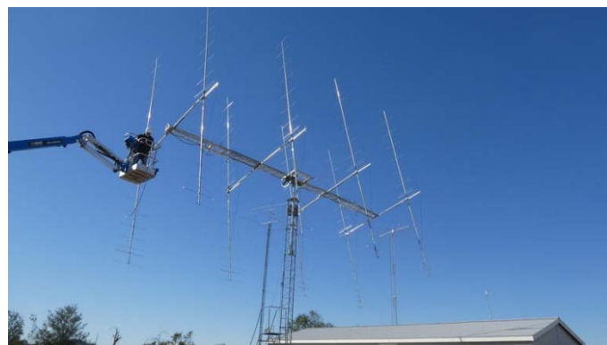
Ned, AA7A (in the bucket) building an EME antenna array for a remotely controlled 2-meter EME station in DM32. The station should be active soon! (Photo provided by Ned Stearns, AA7A)
